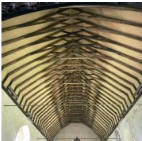
Refurbished roof interior, June 2000.
